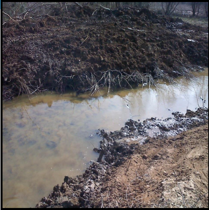
Backfill and rebuild streambank
