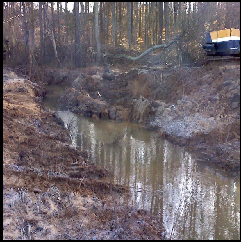
Divert creek away from work area
