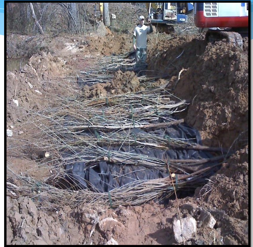
Cover with Geo-Textile Fabric Add more Willow Cuttings
