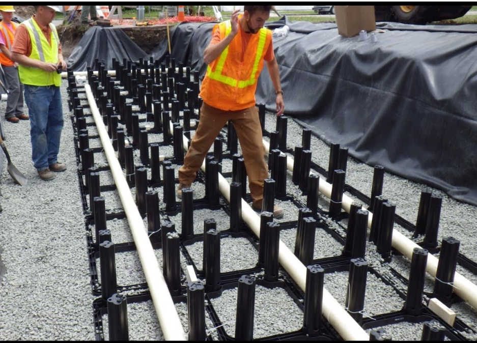
First layer of frames and underdrains...
