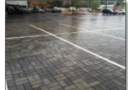
Permeable Pavers Urban Market at Howell Mill
