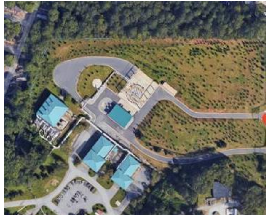
South River Water Reclamation Plant
