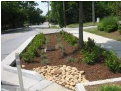
Stormwater Bump-out Whitehall Terrace
