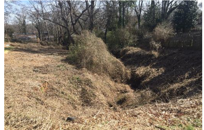
Sewer lines typically follow natural drainage ways
