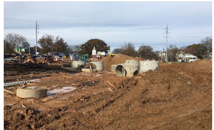
Cook Park regional stormwater project
