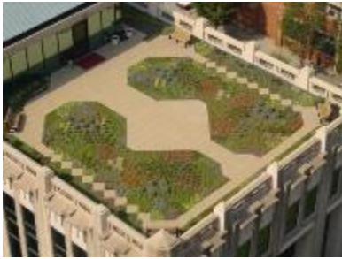
Green Roof City Hall
