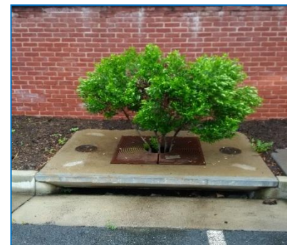
Filterra Box Biofilter
