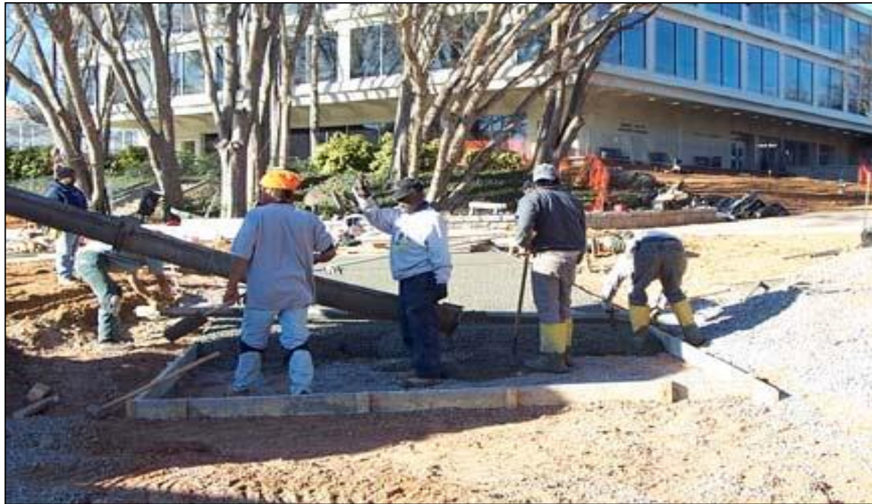
D.W. Brooks Mall, Phase II Construction
