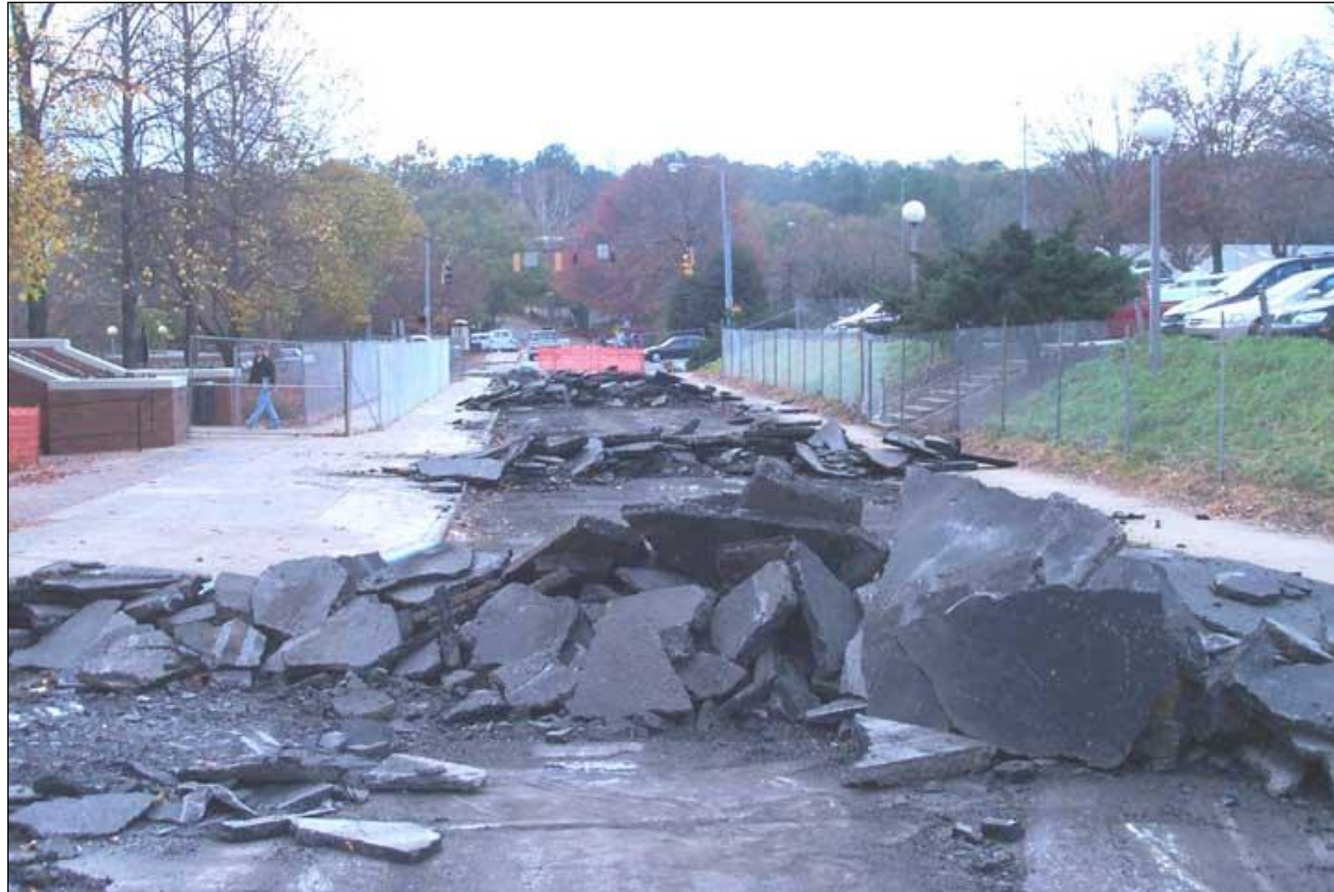
Demolition of Asphalt
